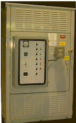
480 Volt, 400 kvar, 5<sup>th</sup> Harmonic Metal-Enclosed Filter Assembly
