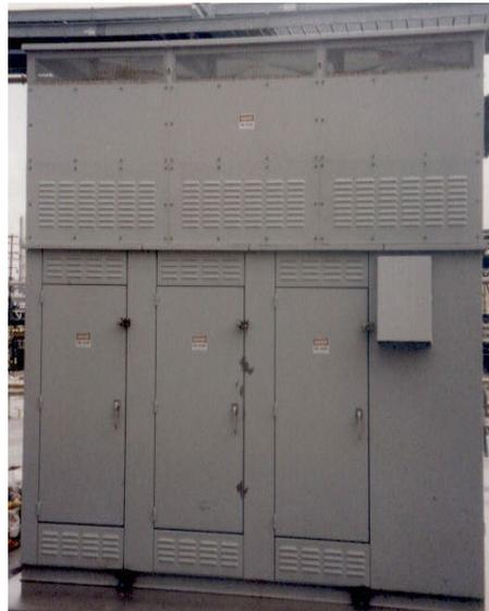
13.8 kV, 3.5 Mvar, 11<sup>th</sup> Harmonic High-Pass Filter Bank with Enclosed Resistor on Top
